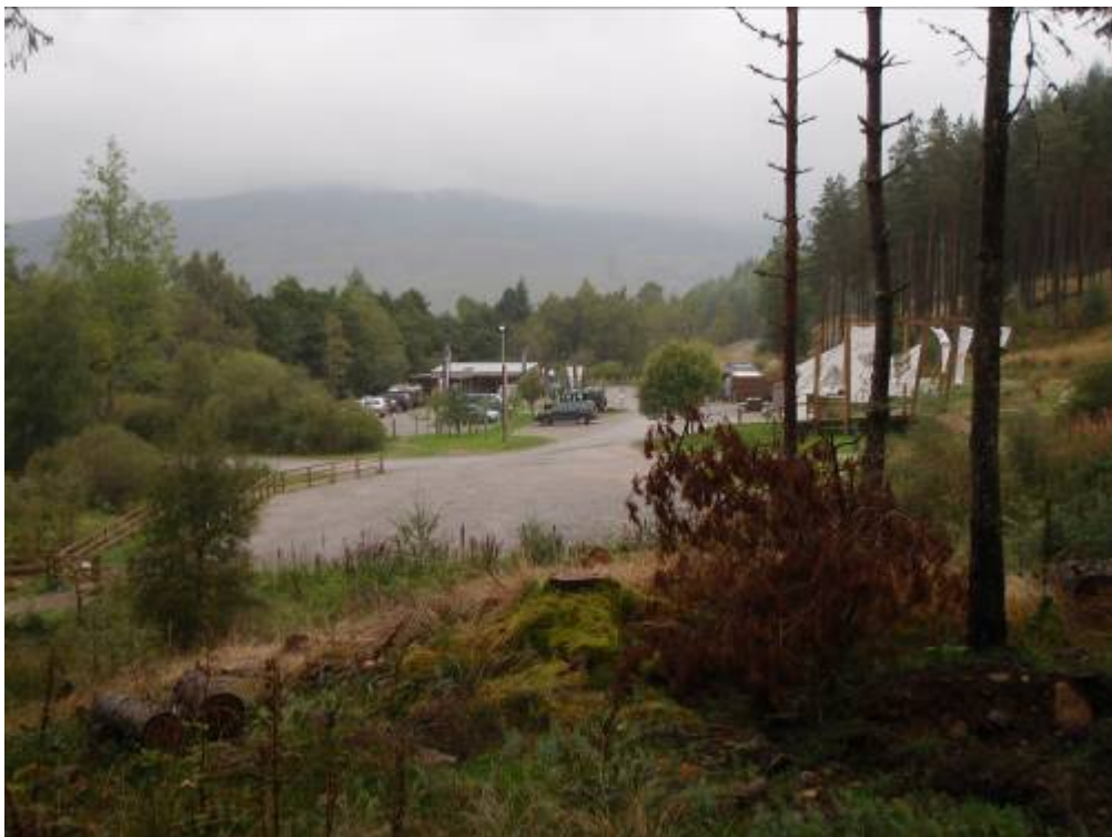
Fig.1 The existing Wolftrax facilities (The site in the foreground)
